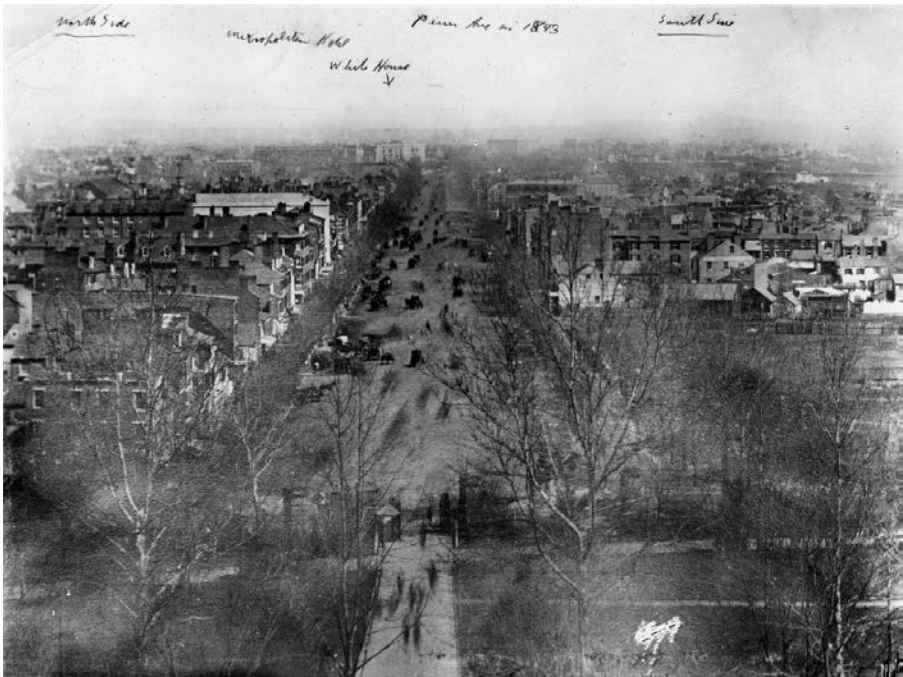
Figure 2.7. View from the Capitol, looking northwest along Pennsylvania Ave. Taken ca. 1843 by W. C. Handy. (Historical Society of Washington, DC, Photo Archives.)
